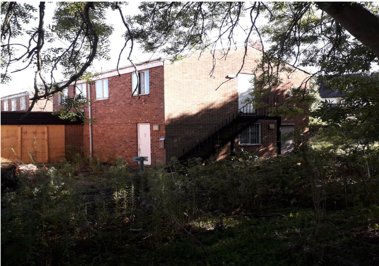
Side elevation of application building
