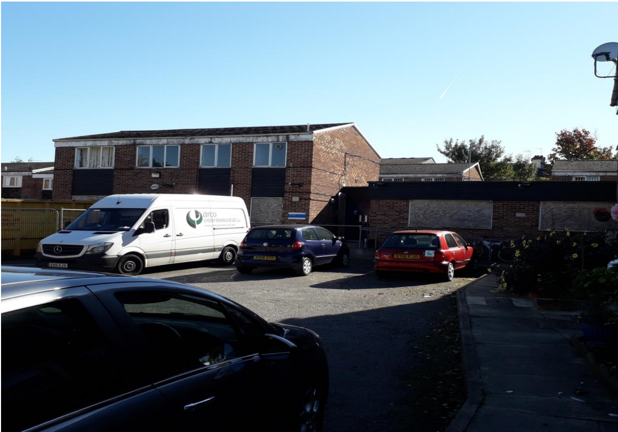
View of application building
