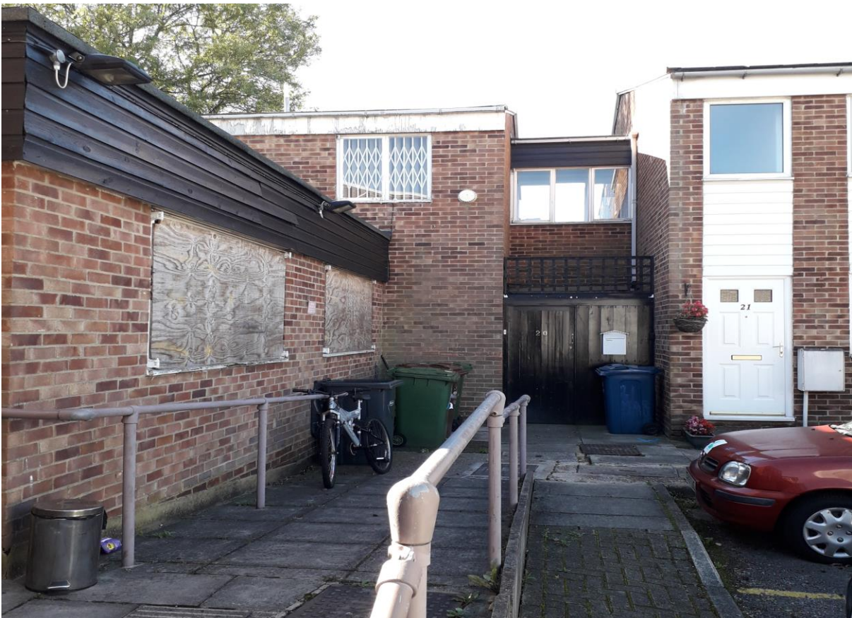
Boundary between application property and neighbouring residents
