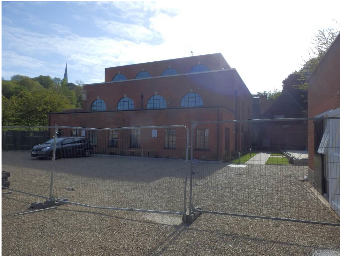
Western elevation of the property
